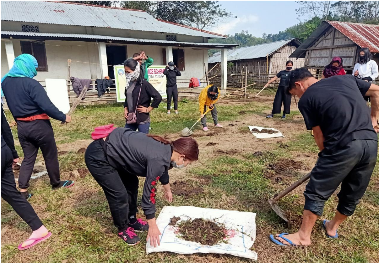
Levelling of School Compound
