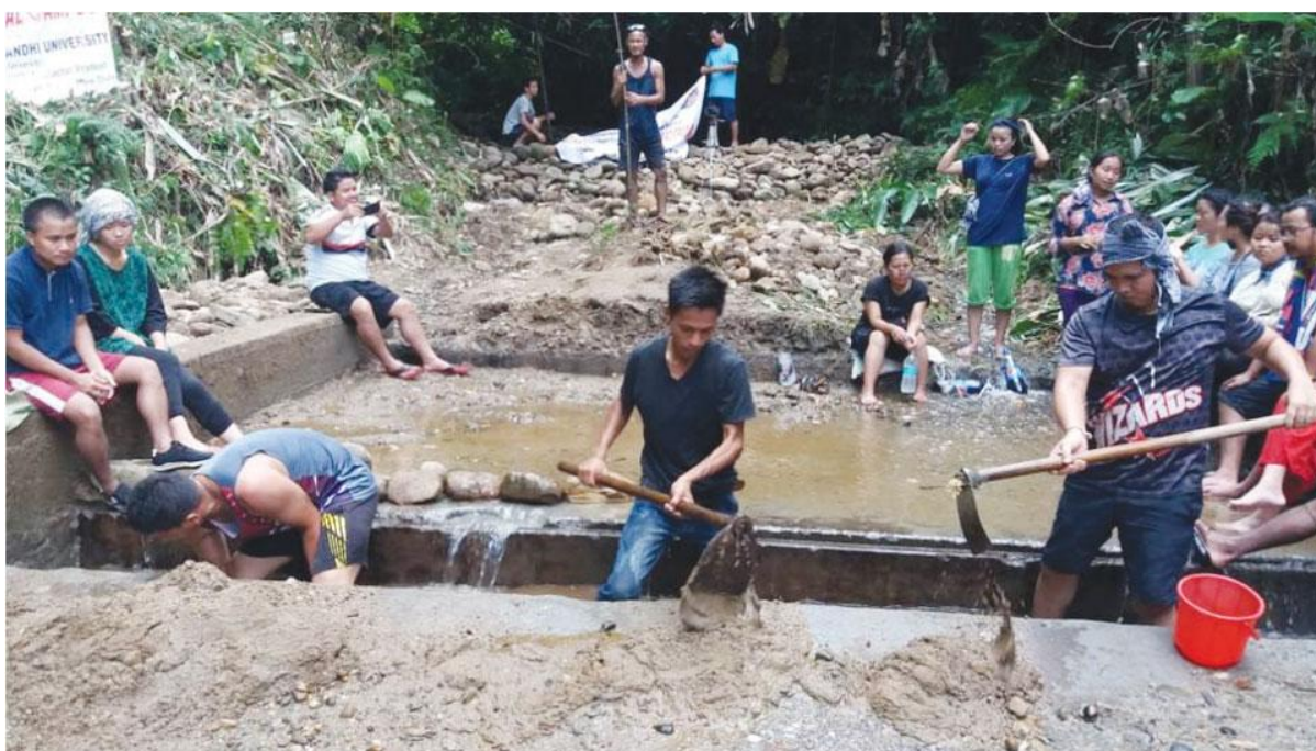
Clearing of Drinking Water Source of Tumru Village
