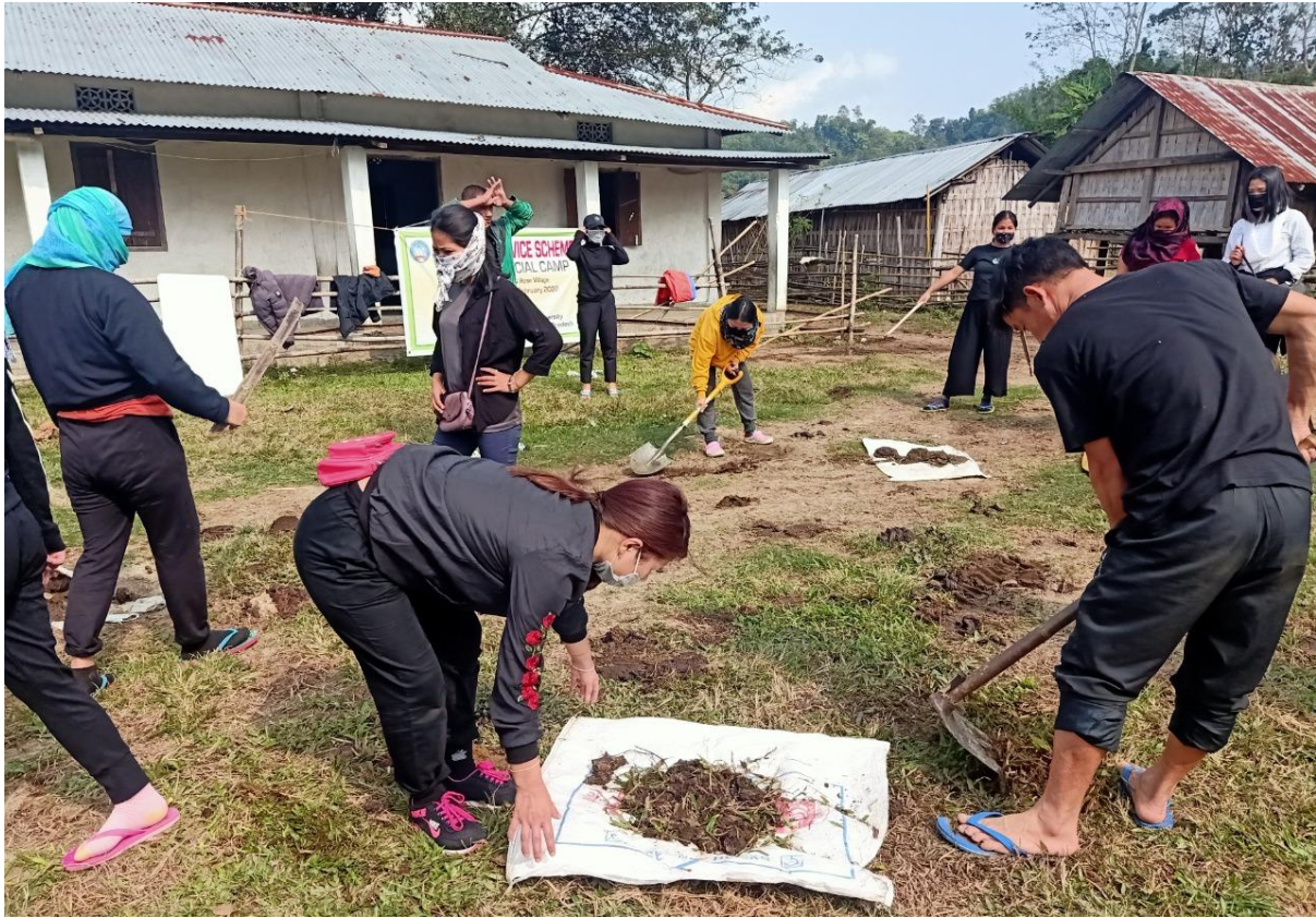
Levelling of School Compound
